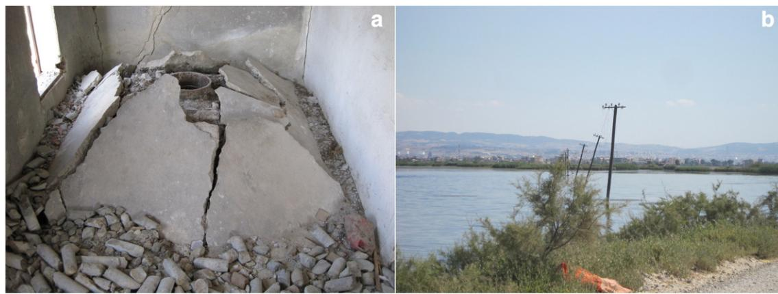
**Fig. 3.** Failures at Kalochori region resulted from the subsidence phenomena. a) Pipe upheaval, b) Damages at the Electricity Network. The photographs were taken in July 2012.
