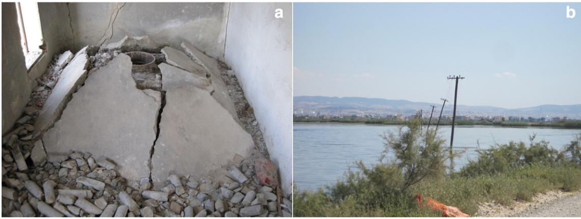
Fig. 3. Failures at Kalochori region resulted from the subsidence phenomena. a) Pipe upheaval, b) Damages at the Electricity Network. The photographs were taken in July 2012.
