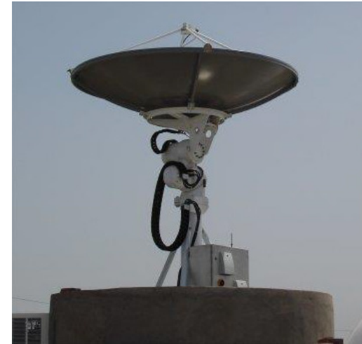
IAASARS/NOA X-/L-band Acquisition station
