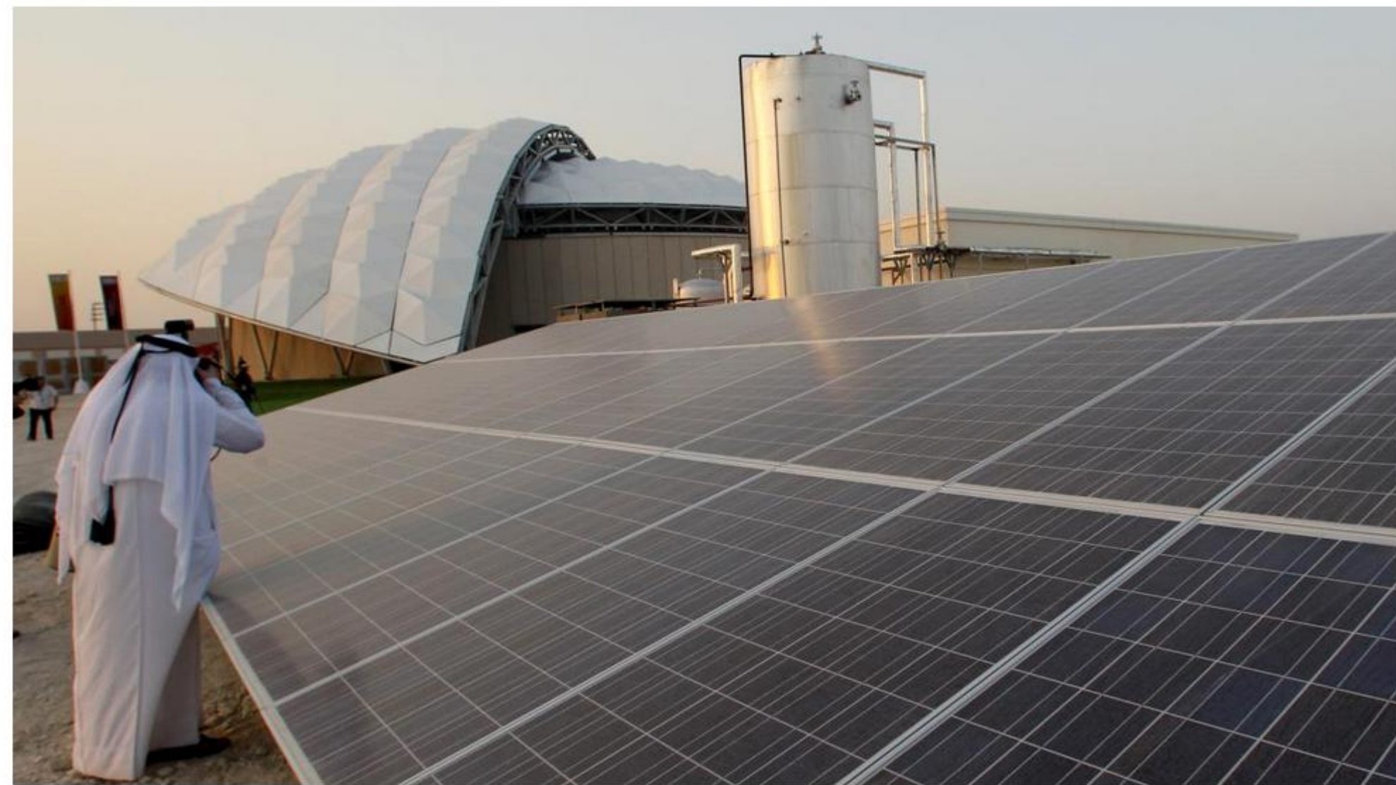
The efficiency of some panels could decline by 30 per cent as temperatures in the panels reached 75C FADI AL-ASSAAD/REUTERS
